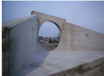
Precast Structural precast Spancrete
