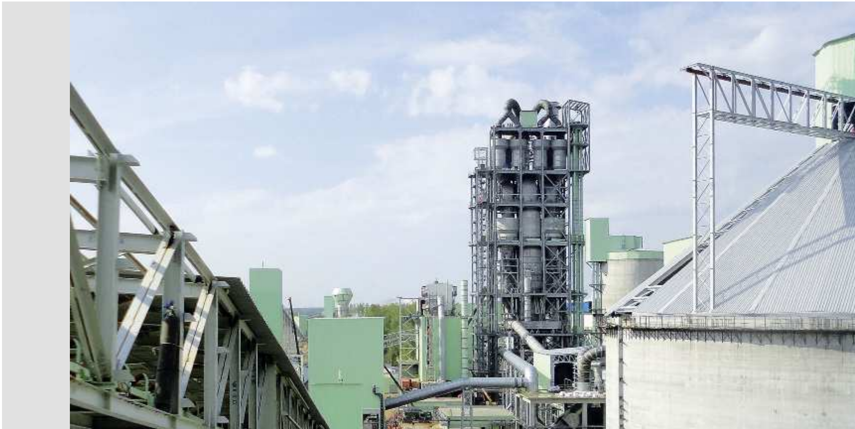
TulaCement plant, Russia
