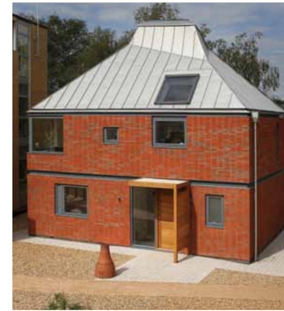
EcoHouse™ – The BRE Innovation Park
