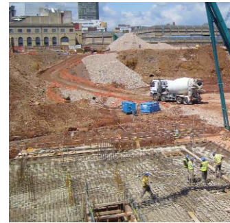
Groundworks at Cardiff St David's.
