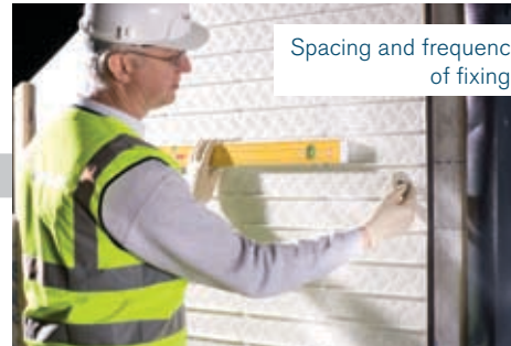
Alignment of backboard
