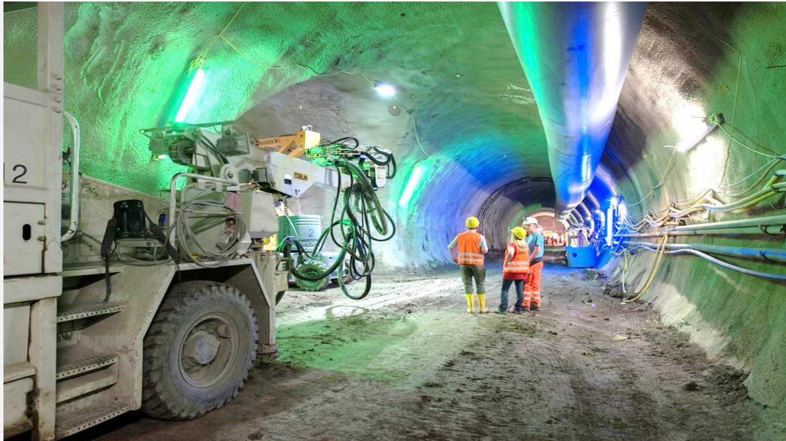
Stuttgart U12 Tunnel Project
