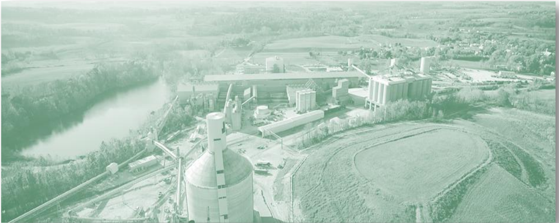
Union Bridge Cement Plant / MD, USA
